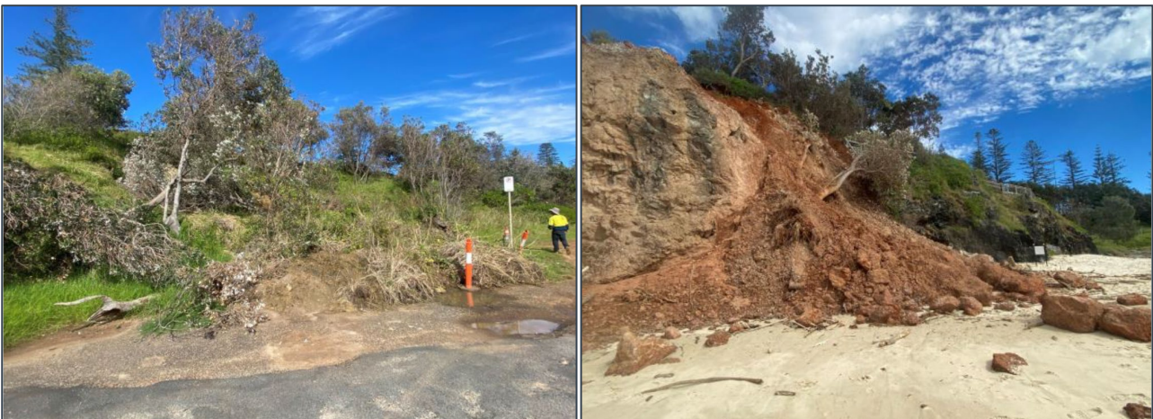
Following heavy rainfall in March 2021 landslips occurred at the rear of the Town Beach car park (left) and at South Oxley Beach (right) (date: 22/04/2021; source: Regional Geotechnical Solutions (2021) March 2021 Flood Event Landslides in Port Macquarie LGA – Parks and Recreation Assets Initial Geotechnical Assessment)
